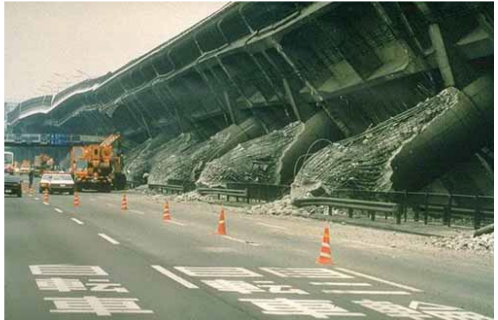
Hanshin Expressway Bridge after Kobe earthquake, Japan, 1995.
