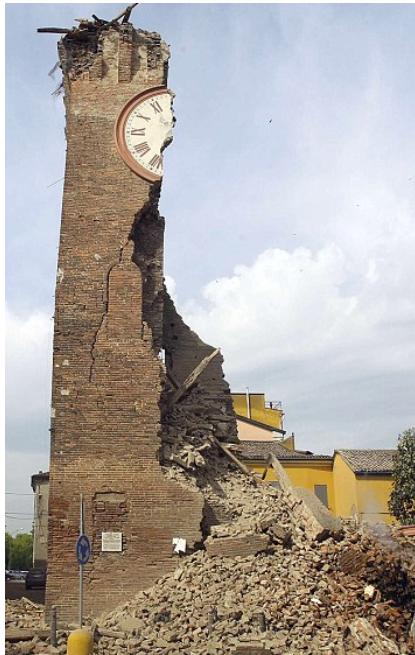
Heritage tower crumbles down in earthquake of Finale Emilia, Italy, 2012.
